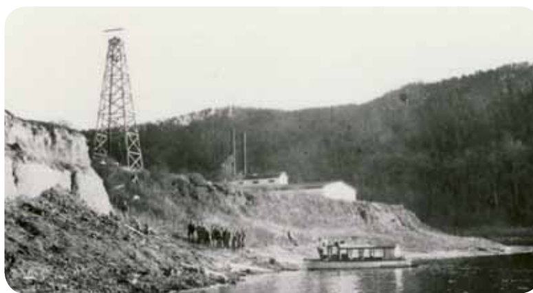
ALBERTA SALT COMPANY'S HORSE CREEK SALT PLANT
