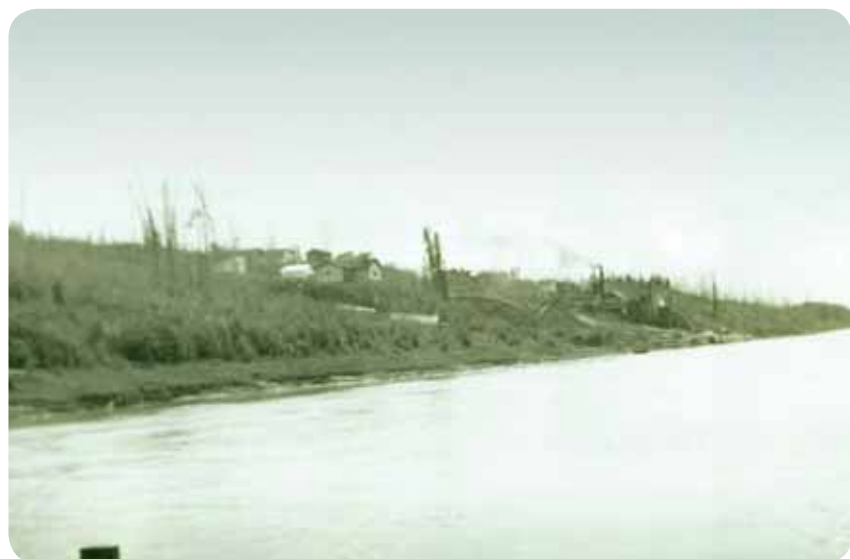
FITZSIMMONS BITUMOUNT OIL PLANT SEEN FROM THE ATHABASCA RIVER, LOOKING SOUTH.
