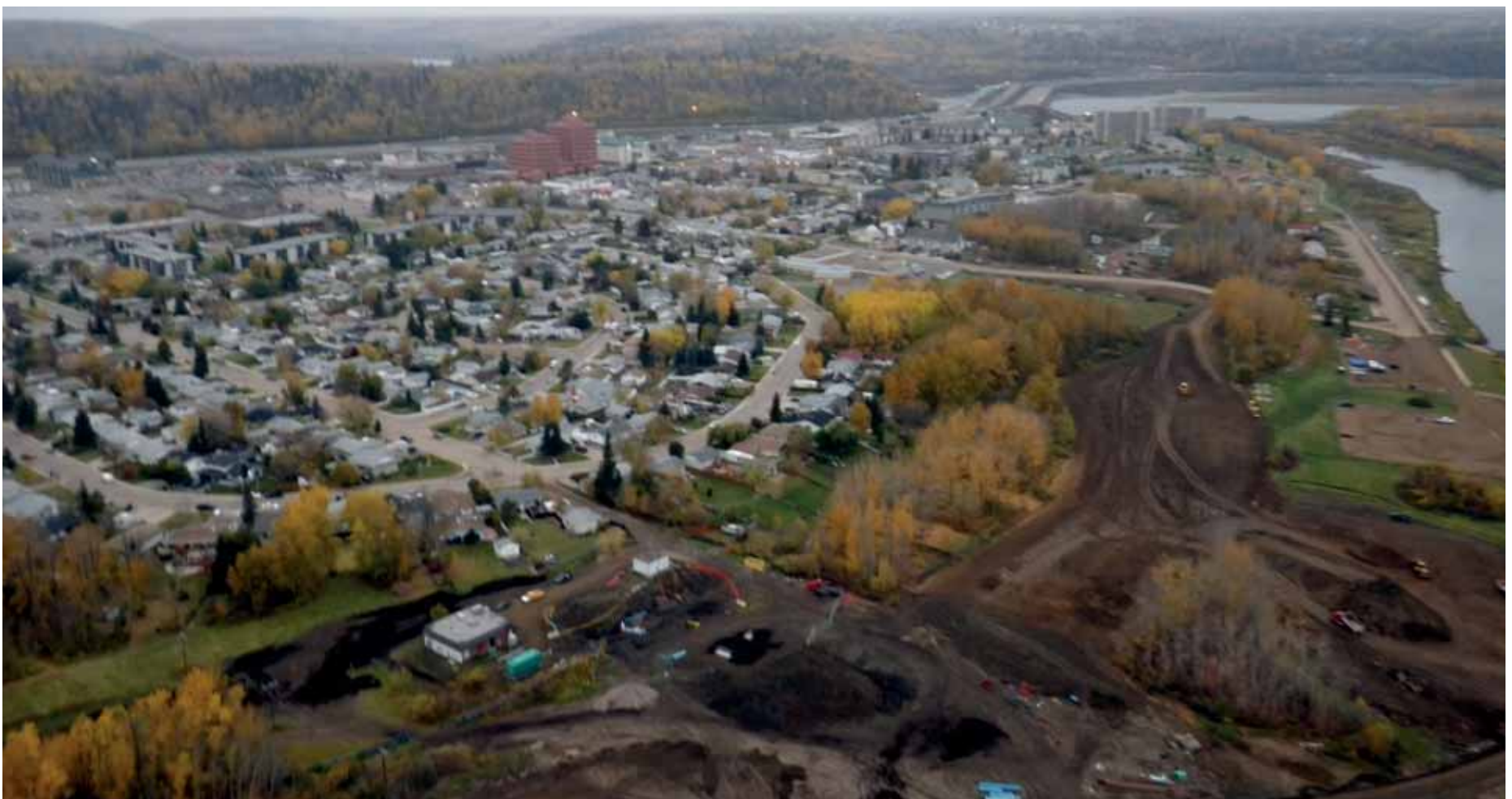
FORMER NORTHERN EDGE OF FORT McMURRAY LOOKING NORTH, FALL 2011
