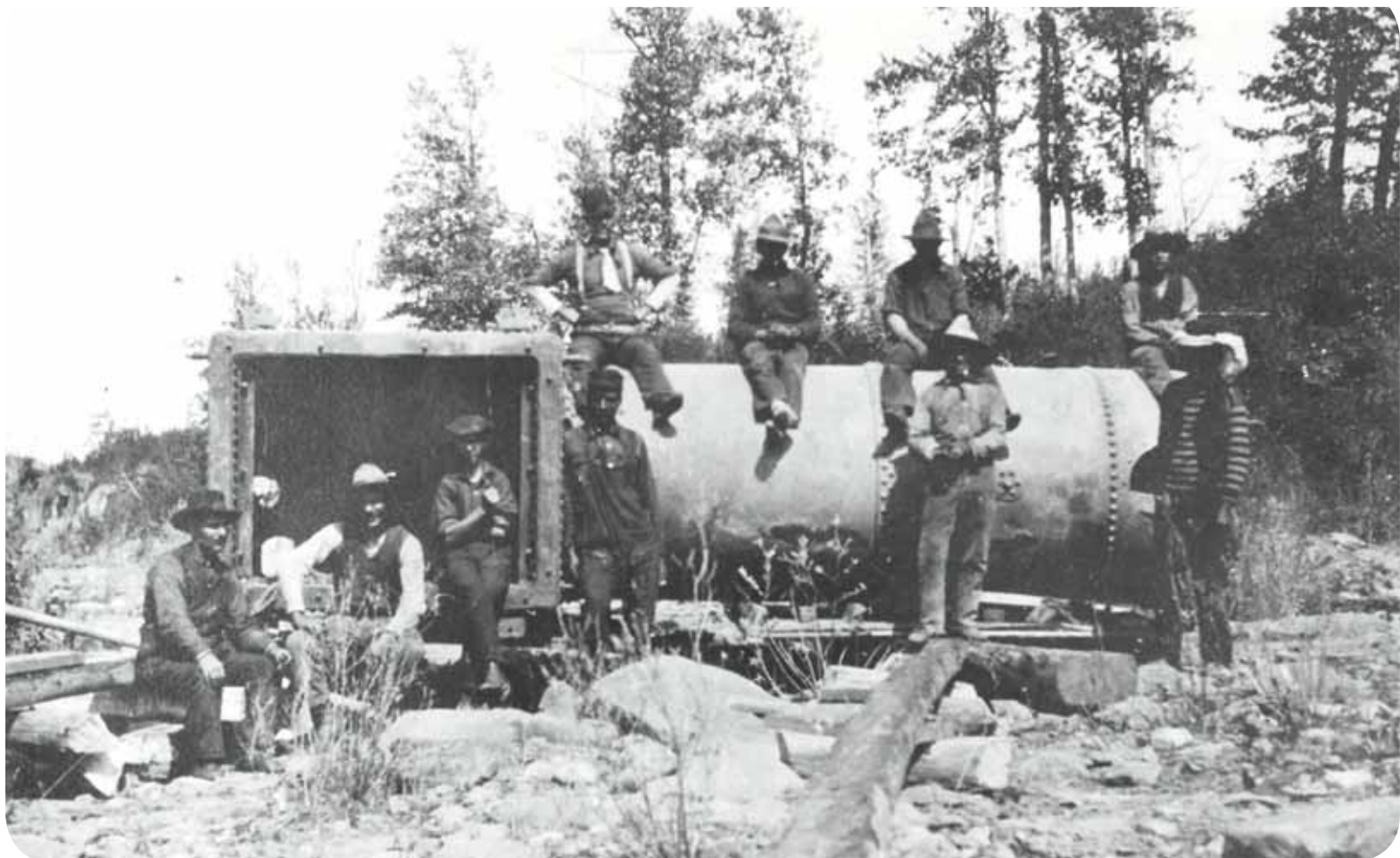
MEN SITTING ON TOP OF A BOILER, CIRCA 1915
