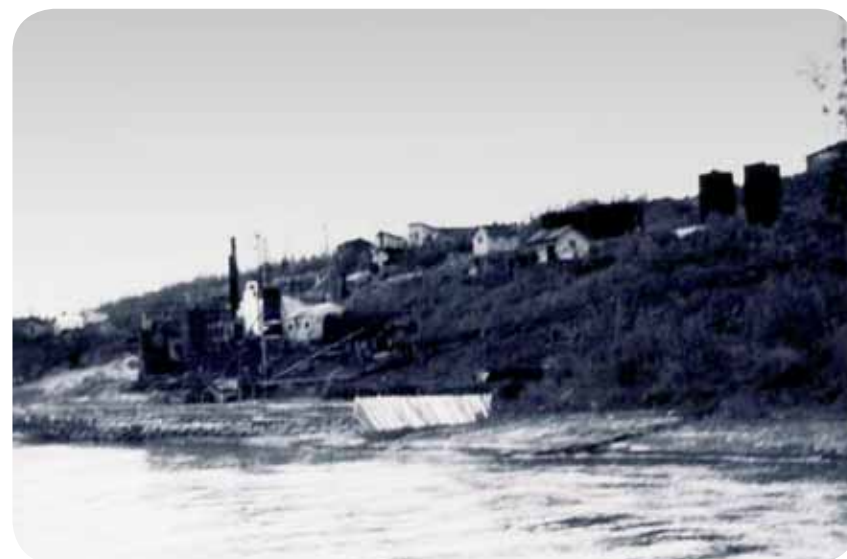
FITZSIMMONS BITUMOUNT OIL PLANT SEEN FROM THE ATHABASCA RIVER, LOOKING NORTH.
